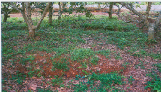
◀ Plate 5. Staggered contour trenches in Cashew Plot
