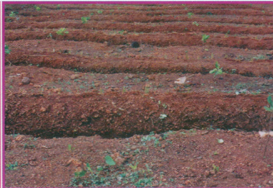
Continuous contour trenches
