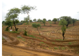
V-ditch contour bund
