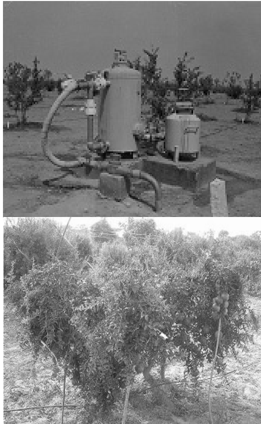
Surface drip system
