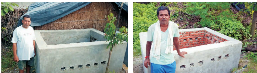
Construction of NADEP Pits during KKA in Udham Singh Nagar
