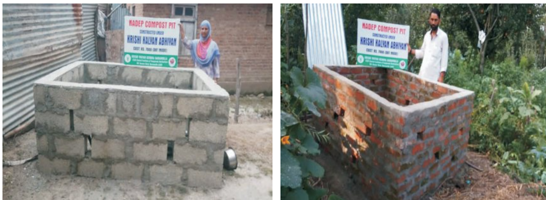
Construction of NADEP pits in district Baramulla
