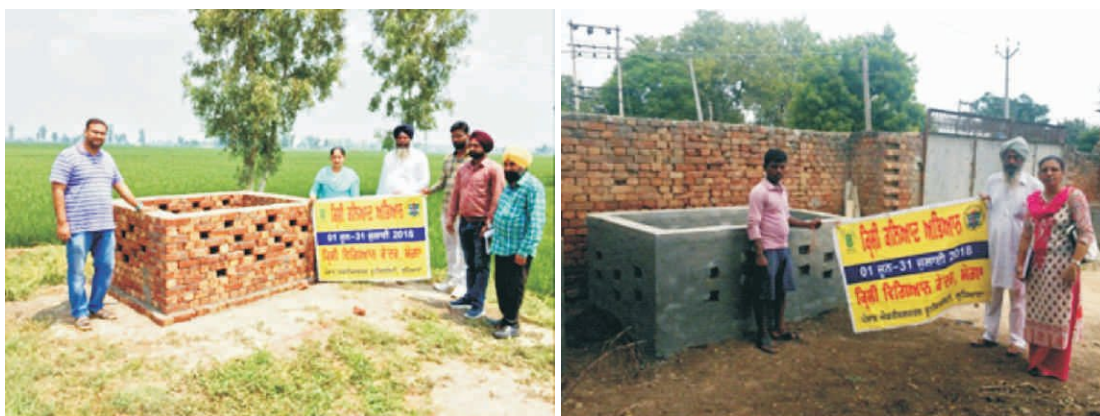
Construction of NADEP Pits in distt. Moga
