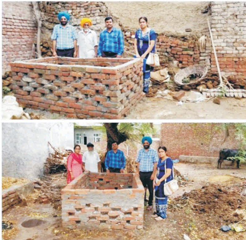
Construction of NADEP Pits in Ferozepur
