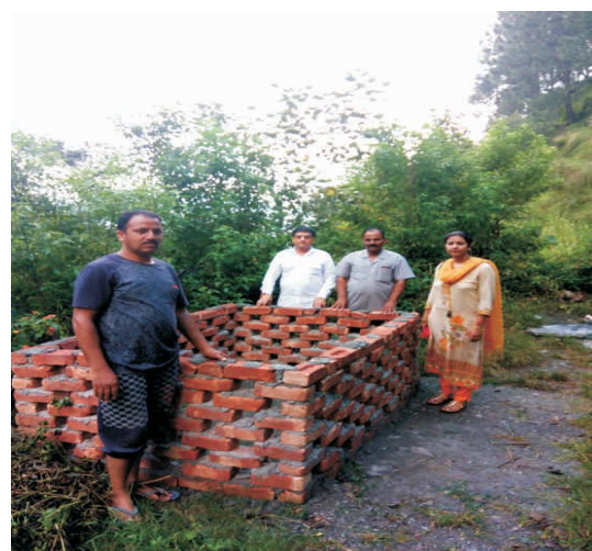
Construction of NADEP Pits in district Chamba
