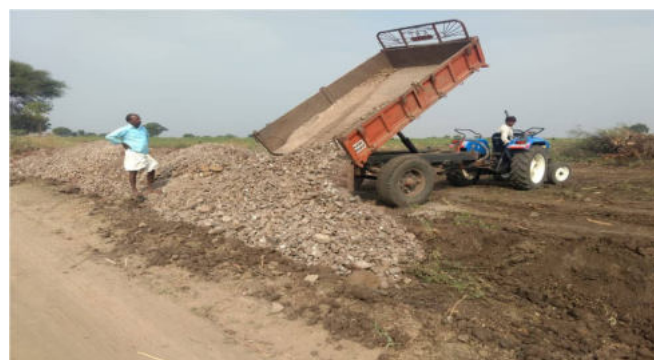
Fig: Bund formation in progress at Kalaburagi
