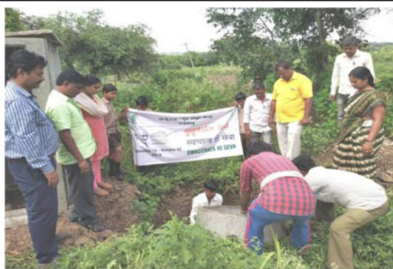
Construction of toilet pit (KVK Belagavi –II)
