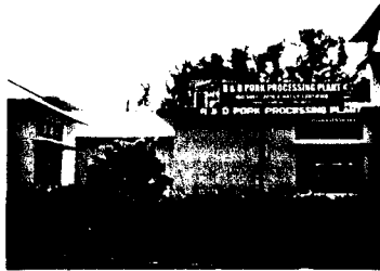
R&D Pork Processing Plant
