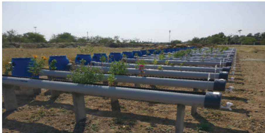
Fig. 2.30. Experimental horizontal sub-surface flow constructed wetland system (HSSF-CWs)
