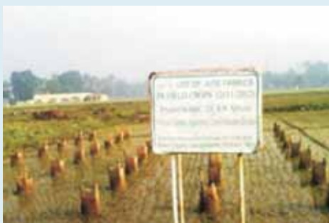
Jute reinforced soil columns in rice field
