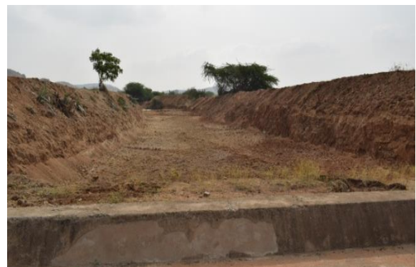
Renovation of Check Dam (Ananthapur)
