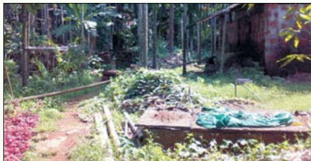
Biogas plant in horticulture based dairy farming
