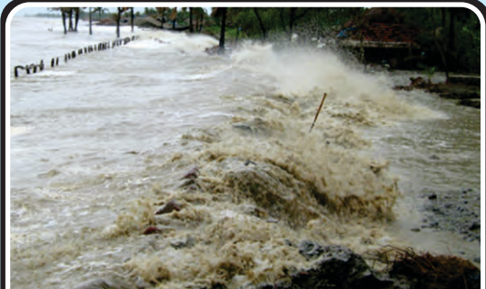
Storm water overtopping the embankment
