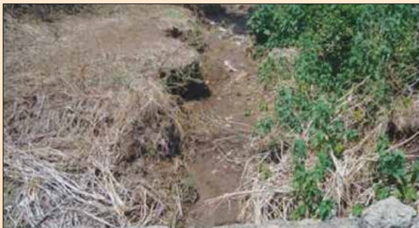
Old Nala (drain) before renovation
