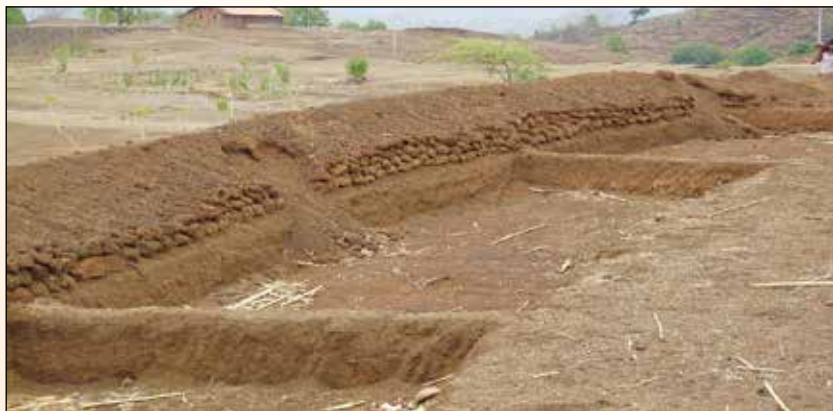
Trenches and compartment bunds
