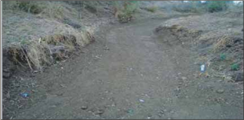
Nala (drain) after renovation
