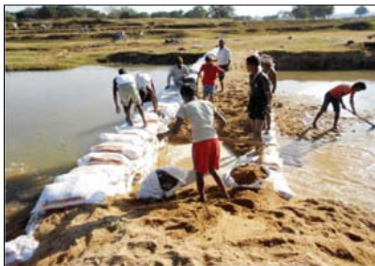
Farmers laying check dam
