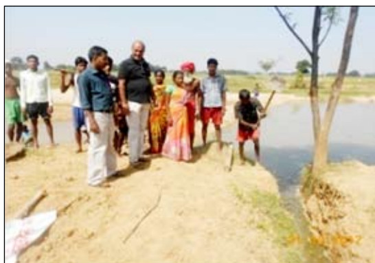
Diverting water for check dam
