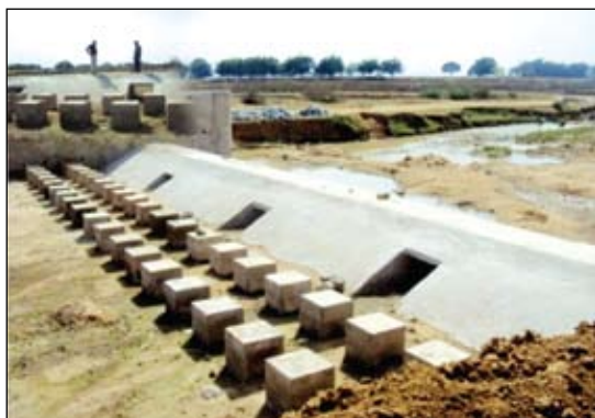
Cement check dam built by district administration
