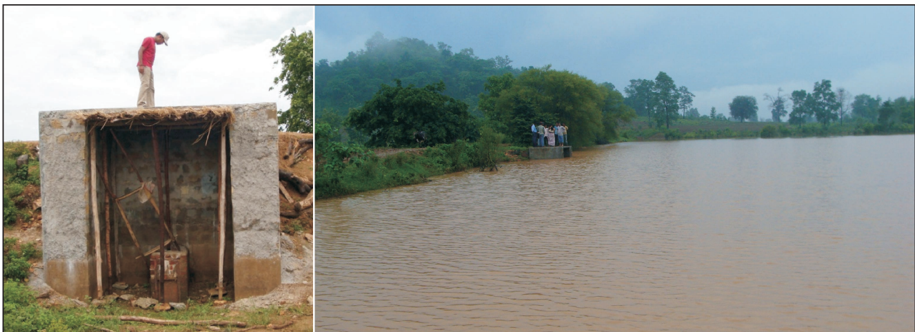
Ippalakunta tank brought back to life by repairing sluice gate (left)
