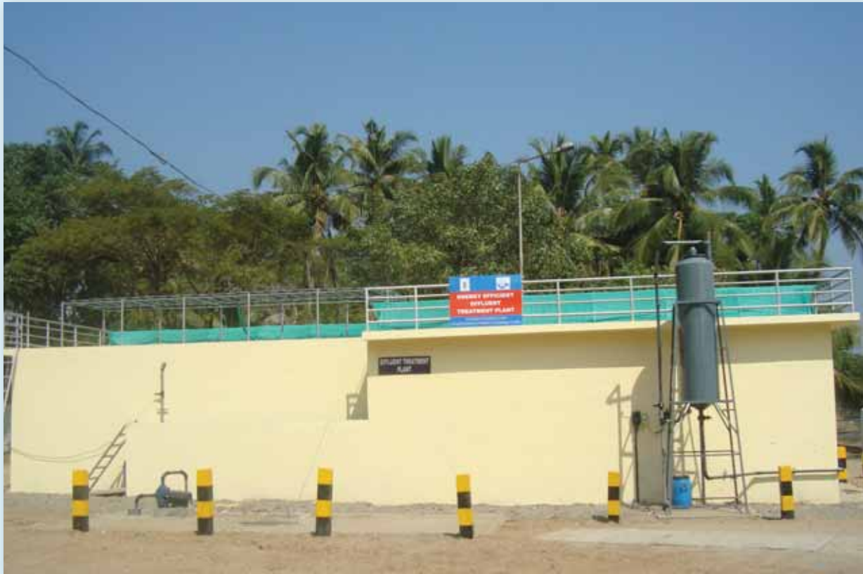
EFFLUENT TREATMENT PLANT
