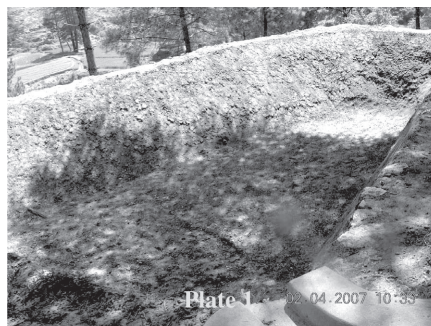
Fig. 4 : Excavation of pit and embankment of the dug out soil
