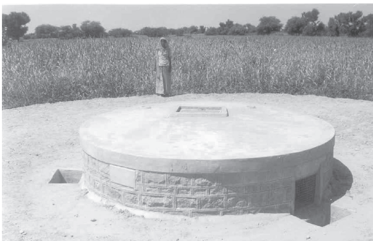
Fig. 8 : Improved tanka of 21 m 3 capacity at Baorali village (Distt. Jodhpur)
