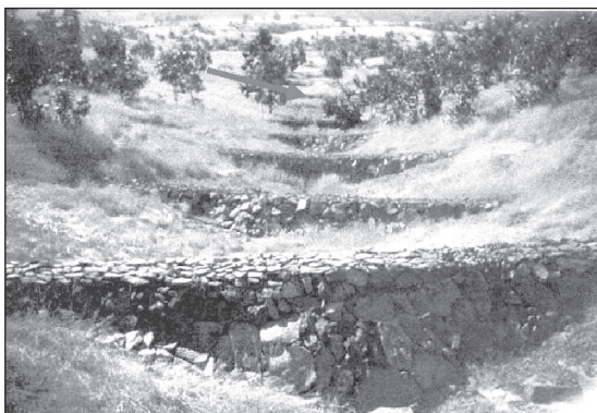
Fig. 18 : Series of loose boulder wall gully checks at Bundi watershed, Rajasthan, India.
