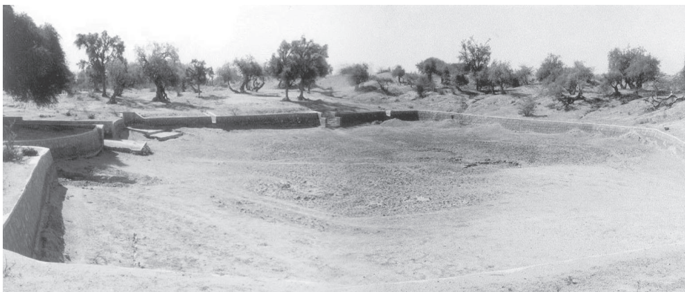
Fig. 9 : Improved nadi with inlet and outlet
