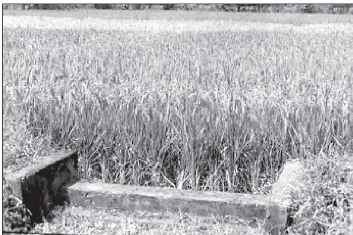
Plate 2 : Brick masonry weir in the downstream side of the rice plot
