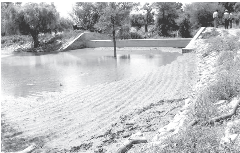
Fig. 10 : Khadin with wastewier at Baorali-Bambore watershed (Jodhpur)
