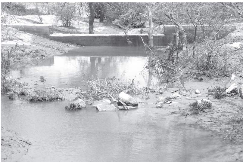
Fig - 6. Check-dam at Beriganga research farm of CAZRI - Jodhpur
