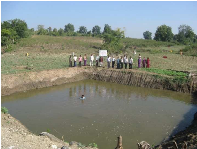
Farm pond dug under NREGS being widened and deepened
