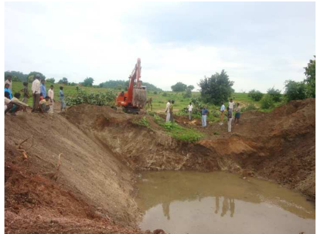
Farm pond dug under NREGS being widened and deepened
