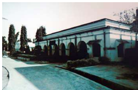
Old Building of CRRI
