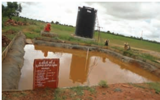
Harvested rainwater in farm pond with cement + soil (1:3) lining
