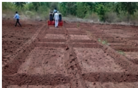
Compartment bunds in kharif
