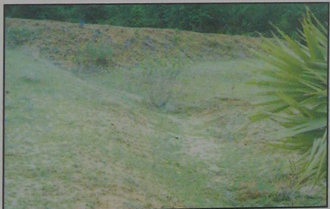
Fig.8.6 Reclamation of gully by constructing percolation pond in upstream of gully
