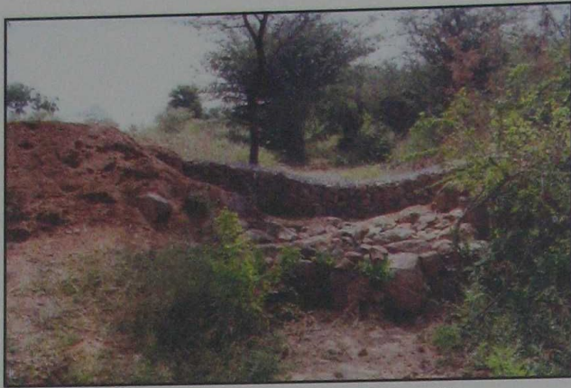
Fig. 7.5 Gabion structure in a gully
