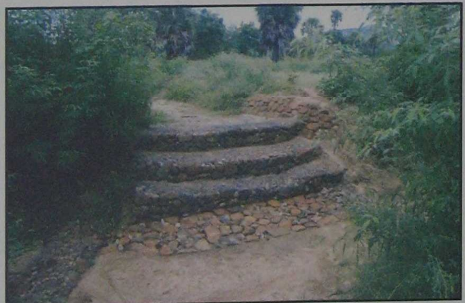
Fig. 7.4 Gabion drop structure
