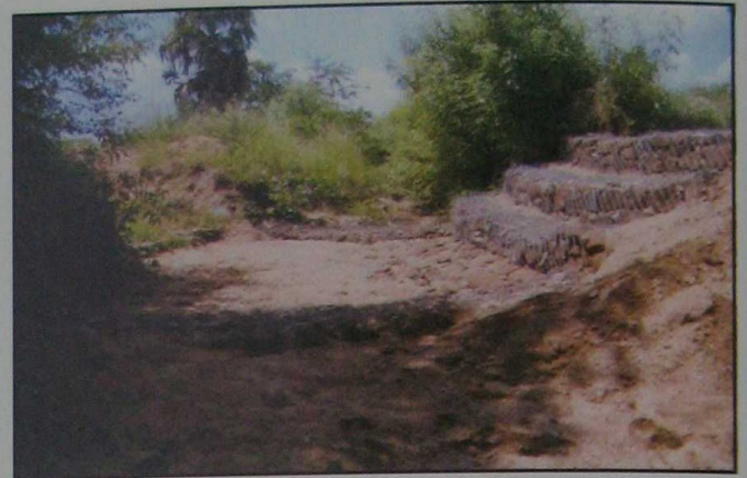
Fig. 7.6 Cascading gabion structure
