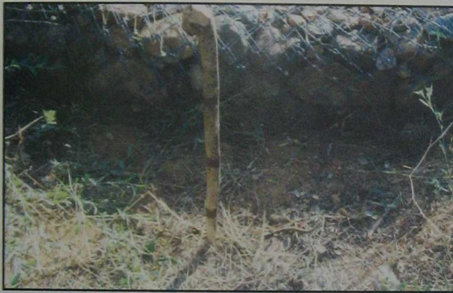
Fig.8.3 Graduated wooden peg at upstream side of gabion structure
