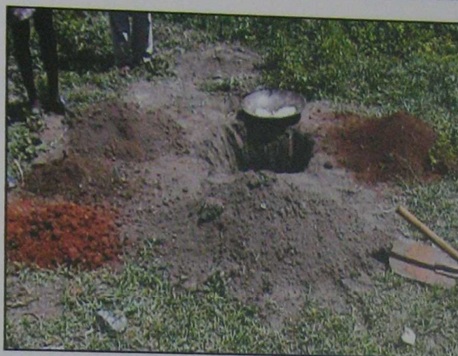
Fig.10.6 Removal of soil layer from pit
