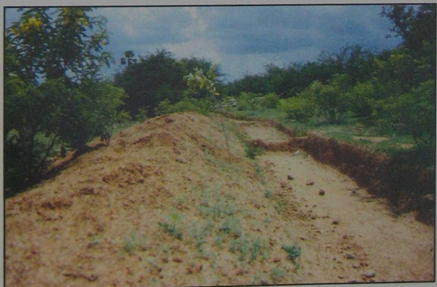
Fig. 7.1 Diversion channel in watershed area
