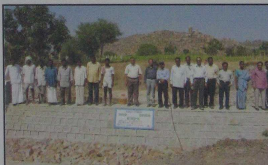
Check Dam at Chowderpalli in Mahaboobnagar
