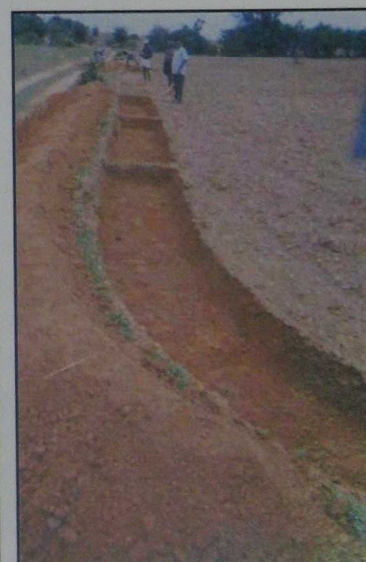
Trench-cum-bund in Tiptur cluster
