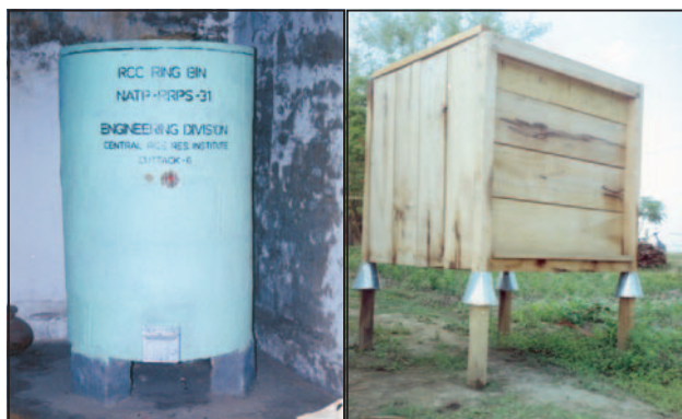
Improved paddy storage structures : RCC Ring bin in Cuttack district (left) and rat proof wooden storage structure in Imphal district (right)
