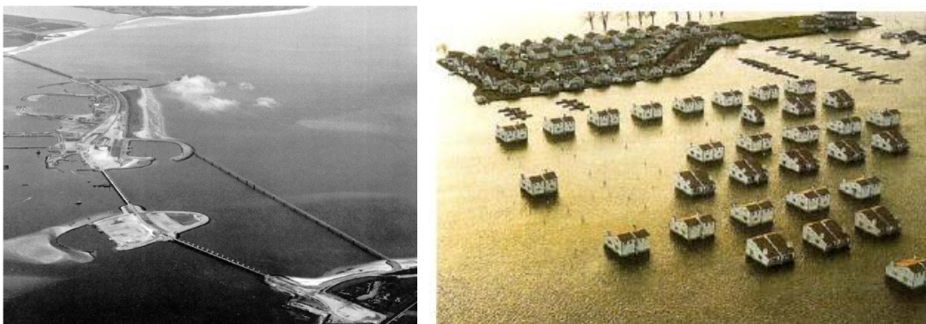
Figure 3 Storm surge barrier at Oosterschelde (left) and floating neighbourhood in Netherlands
