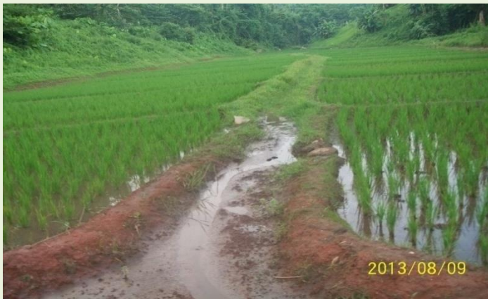
Improvement of existing of Paddy field by constructing Bunds
