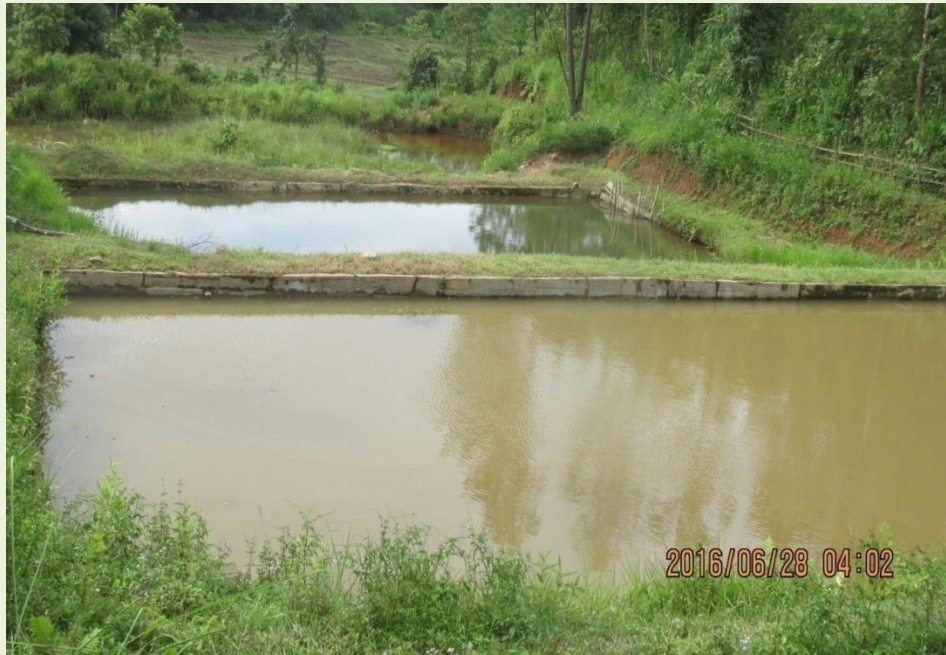
Community Water Harvesting Structure at Umsarang Village under Umsarang IWMP-I GPS Reading: N-25°43'08.1" :: E- 92°01'37.8"
