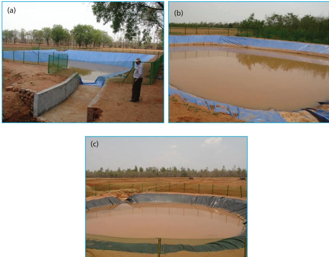
Fig. 12(a,b&c) : Different shapes of farm ponds with Silpaulin and HDPE lining
