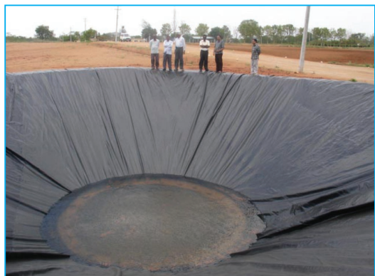
A complete view of lined farm pond with HDPE film
