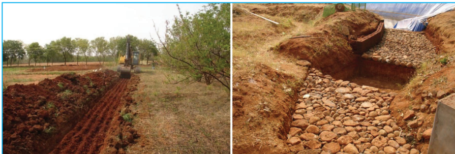
Fig 16. A view of inlet channels and stone pitching in spillway
