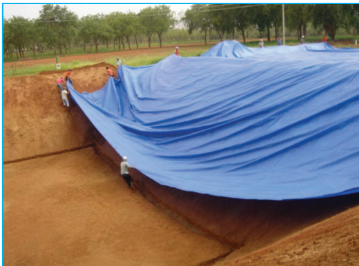
Spreading of silpaulin plastic film
