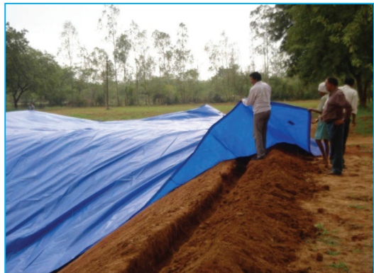
Anchoring of the lining film on top and soil filling
