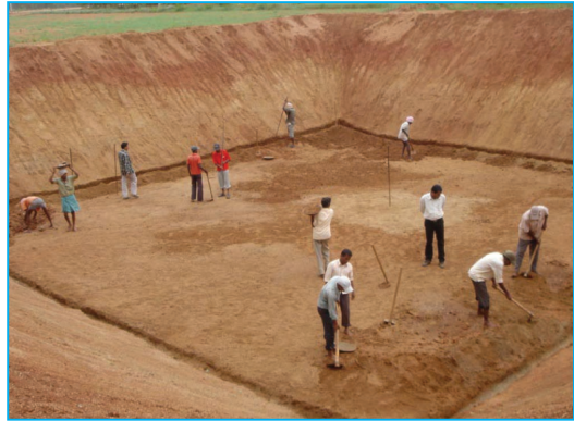
Square: Making trenches for anchoring lining plastic film
