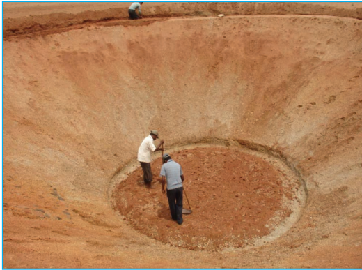
Inverted cone: Making trenches for anchoring lining plastic film
