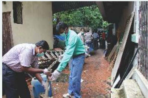
Fig. 13.8 Removing debris and scrap equipment from the QEID
