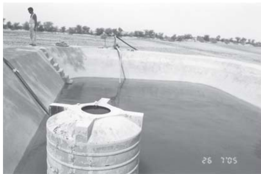
Neutralization of RSC water through gypsum tank for sprinkler irrigation
