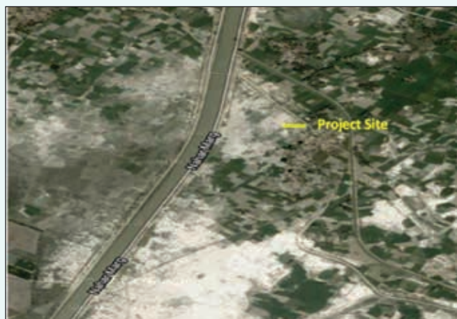
Aerial view of Project Site (Patwakhera, Lucknow)
