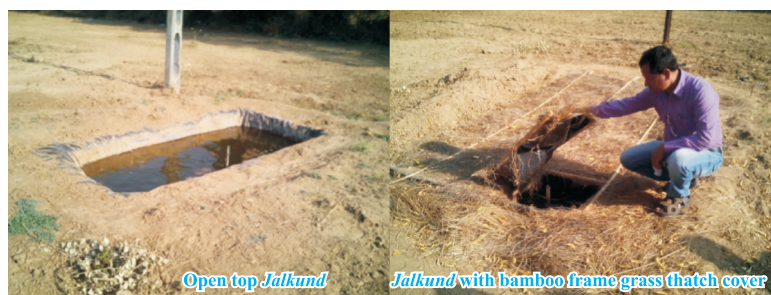
Photo 3.17: Open and bamboo frame grass thatch cover with opening for water removal Jalkund
