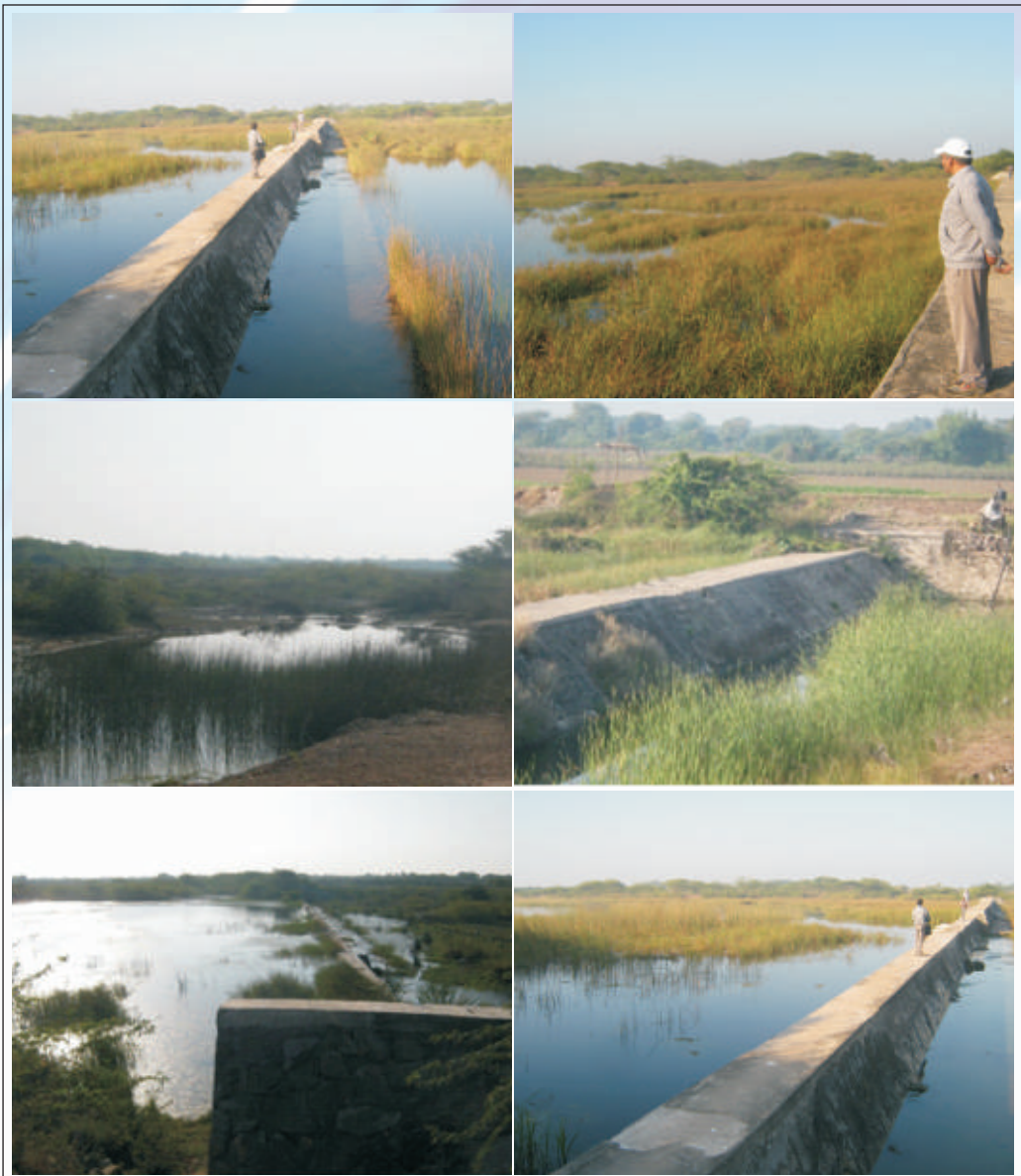
Plate 9: Maintenance status of community check dams at the time of survey
