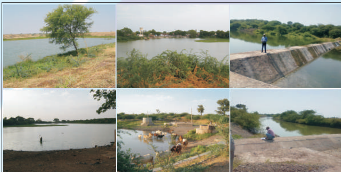
Plate 2: A profile of community based water storage structures (community ponds and check dams) studied
