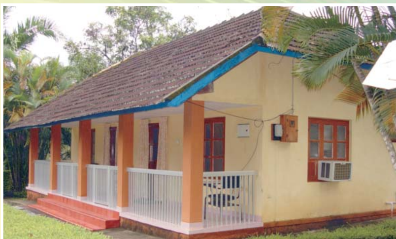
Renovation of guest house at NRCOP-RS, Palode
