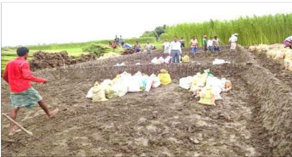
Digging of temporary pond
