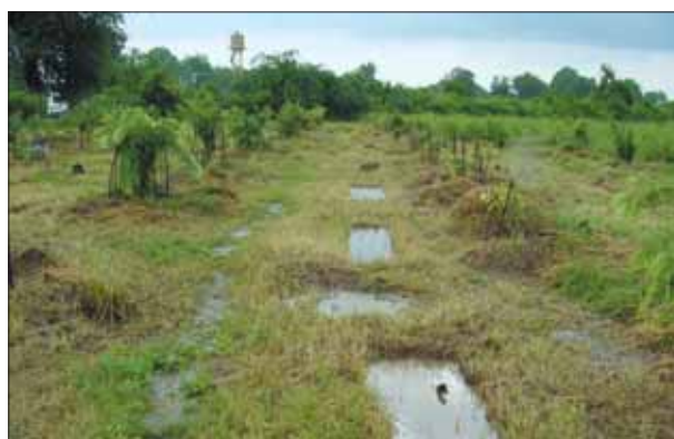
Staggered contour trenching for horti-pastoral land use in medium deep ravines – Kota
