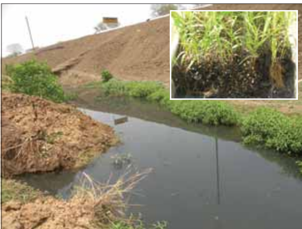
Waste water carrying drain; Inset: Arundo grown in angular gravel media (without soil)
