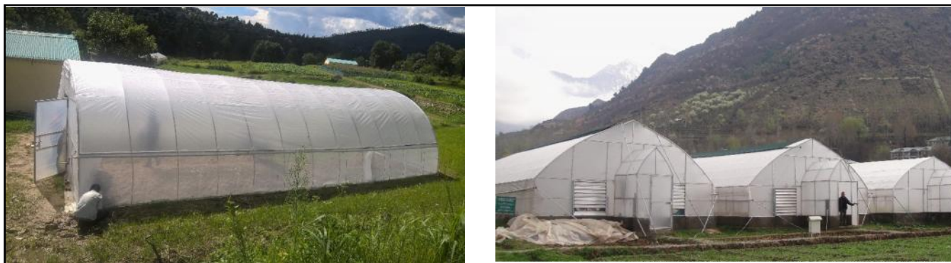
Fig. A and B : Walk-in tunnel/Quonset and Gothic type polyhouses in J & K, Uttarkhand and Himachal
