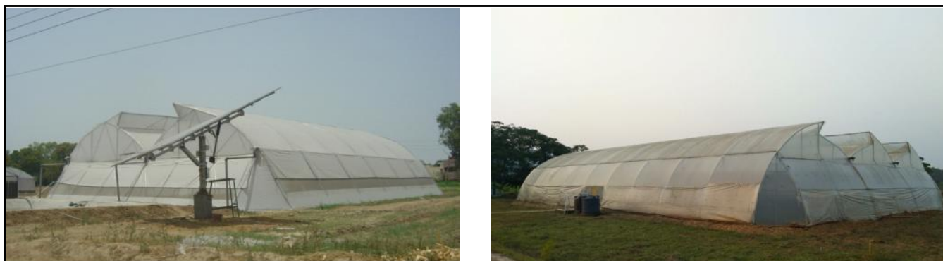
Fig. C and D : Double and Multi-span saw tooth polyhouses of Punjab, Gujarat, Raichur and Rajasthan
