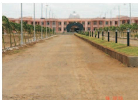
Fig.5: Newly constructed office-cum-laboratory building of NRCP at Kegaon
