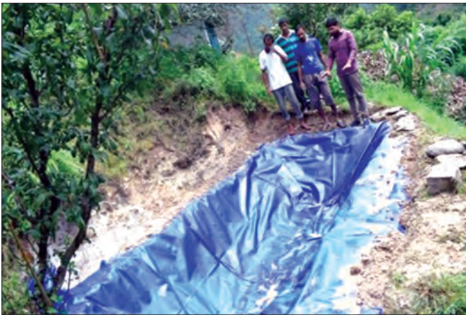
Laying of polyfilm
