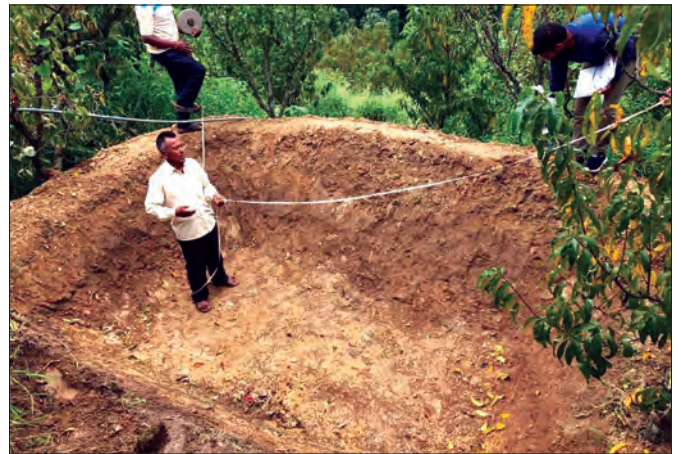
Compaction and measurement of polyfilm
