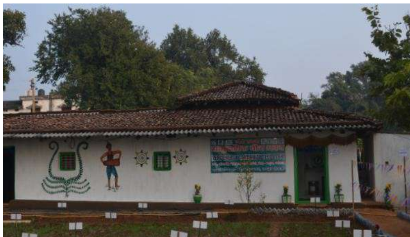
Fig 3. Zero energy low-cost seed bank at Saliyahdih
