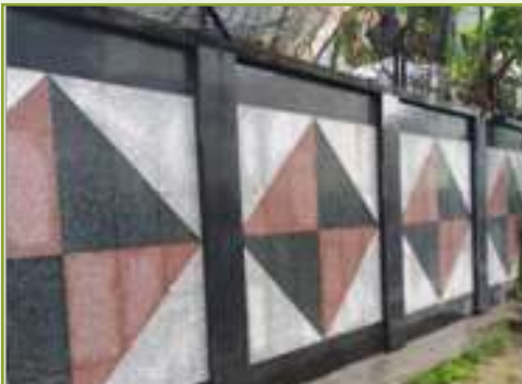
Renovated boundary wall
