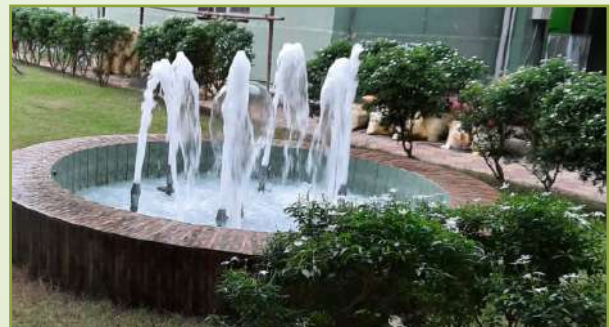
Repairment of fountain in front of Administartive building
