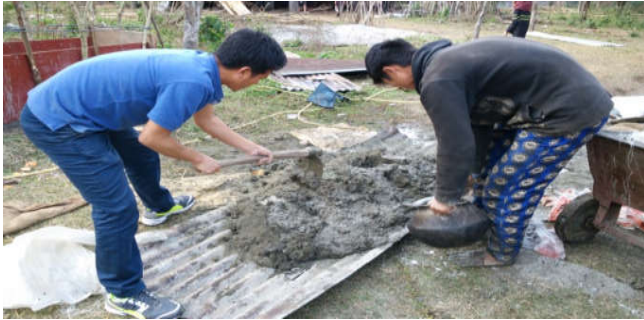
Fig 5 Mix sand, cement and stone gravel, in ratio 4:1:2 respectively
