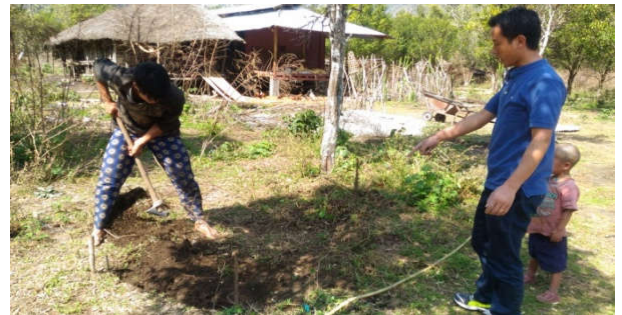
Fig 1 Clearing and measurement of area for earth cutting
