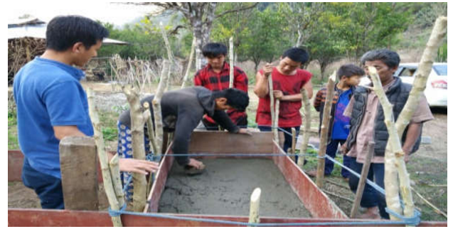
Fig 9 Level it properly using flate wooden material for better licking for Mithun
