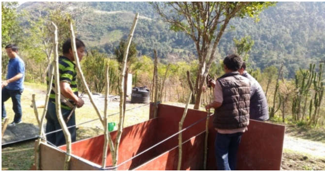
Fig 4 Give support to wooden box with locally available wooden material
