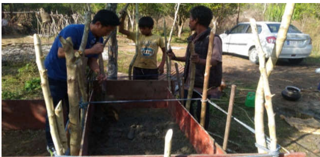
Fig 6 Transfer the mixture into the fixed wooden box & fill up to 2.4ft
