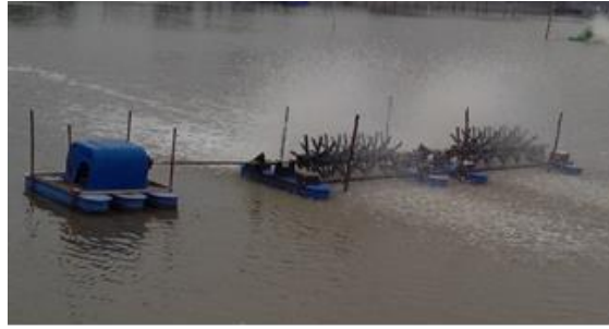
Fig. 3 Spike aerator in shrimp farms
