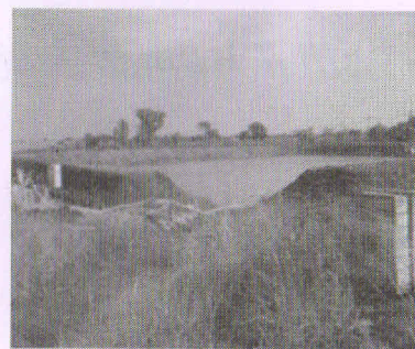
Rain Water Harvesting Pond
