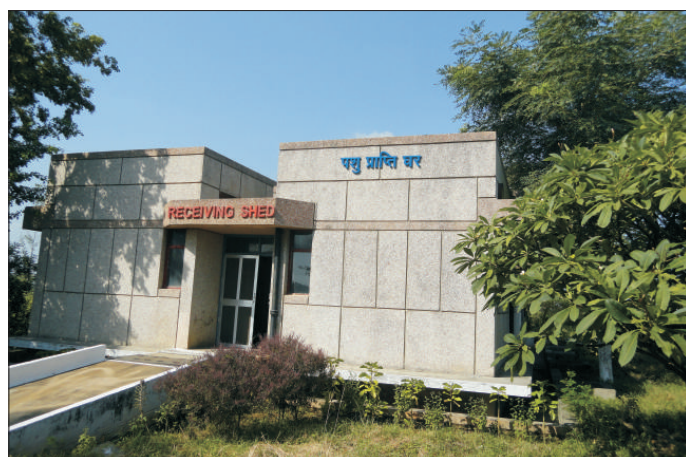
Entry of Receiving Shed
