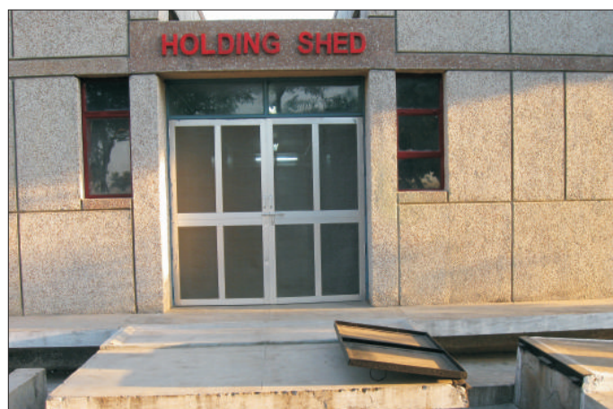
Entry of Holding Shed
