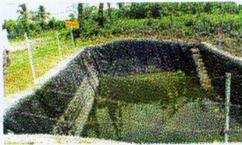
Fig. 24 Rain Water Harvesting in Polythene Lined Pond
