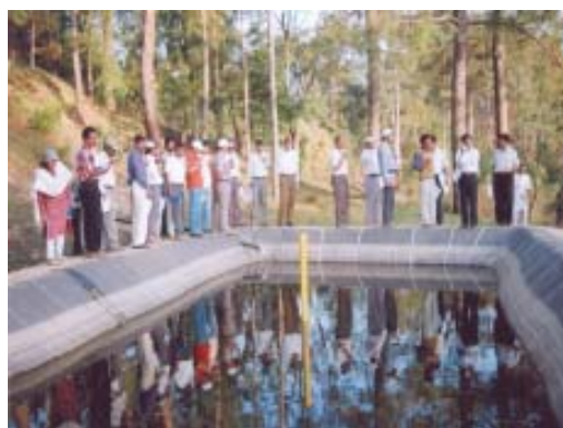
LDPE lined tank for harvesting rain water
