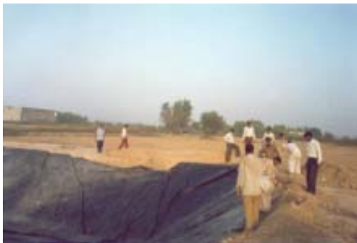
Fig. 6: Burying the side of the Agri-film with soil
