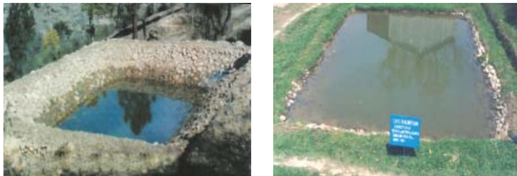
Fig. 10 : LDPE lined with stone pitched tank
