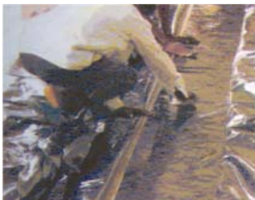
Fig 4a: Cleaning of film before joining
