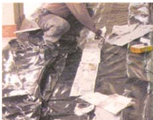
Fig 4b: Teflon sheet or newspaper placed on the film and joining by electric press
