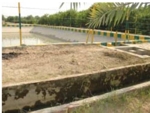
Fig 9: A view of Agri-film lined service reservoir connected with the watercourse
