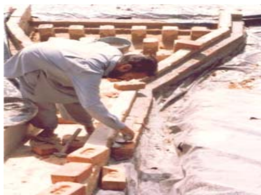
Fig 8: Joining of Agri-film with inlet structure
