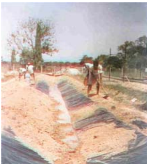
Fig. 11: LDPE lining of water channel
