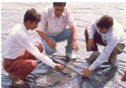
Fig. 5a: Damage of the Agri-film during laying
