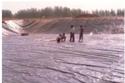
Fig. 7: View of final laying of Agri-film
