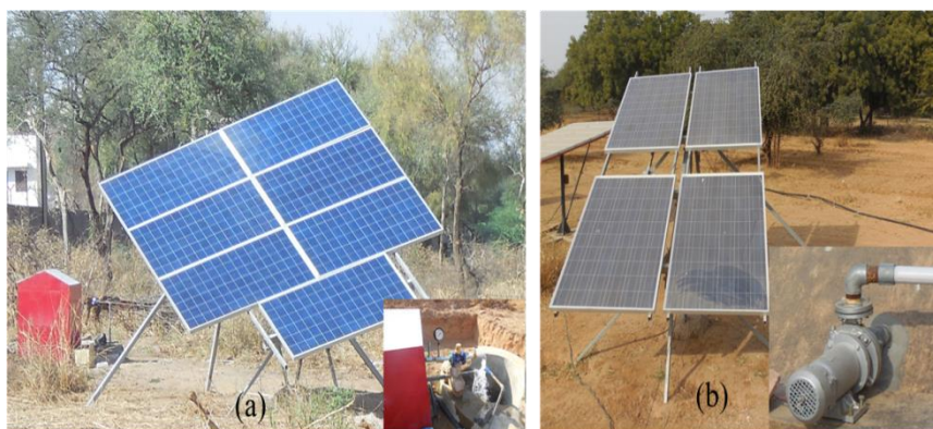
Fig.2. Solar PV pumping system (a) 1 HP AC pump and (b) 1 HP DC pump
