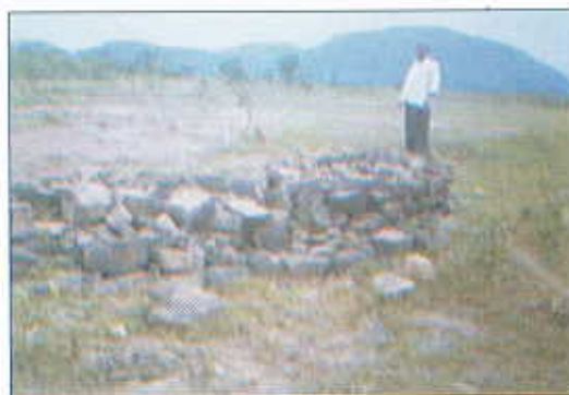
Photo- 25 : Loose boulder structure in the watershed to check runoff and soil loss
