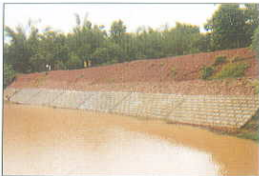
Photo- 20 : Stone patching on the wall of cross bundh
