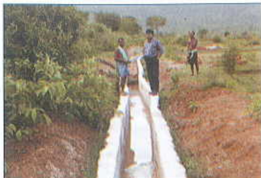
Photo- 24 : Brick made irrigation channel
