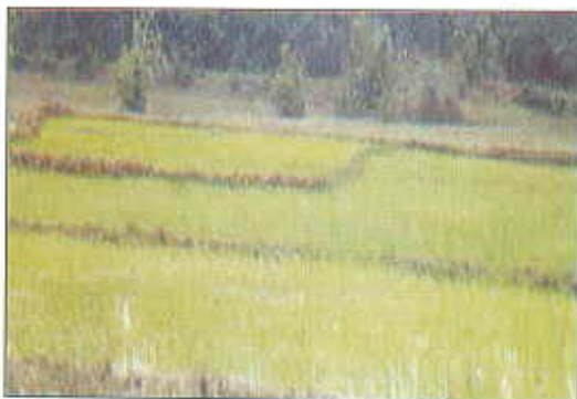
Photo- 21 : Construction of bund around rice field
