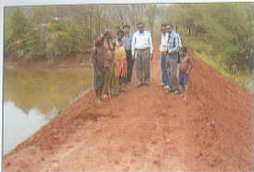
Photo- 19 : Construction of cross bundh
