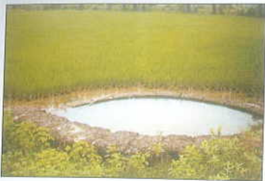
Photo- 26 : Construction of dug well in the corner of the field
