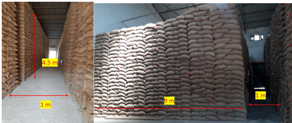
Fig. 3. Stack arrangement of food grain bags inside a conventional warehouse: lengthwise (left); and widthwise (right).
