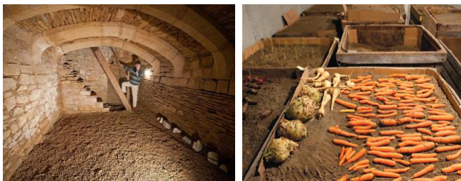
Fig 2 Cellars ventilated storage structures
