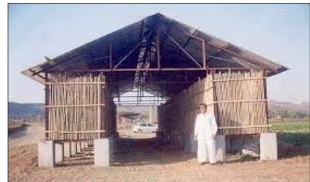
Fig 4 Nasik type ventilated storage structure for onions
