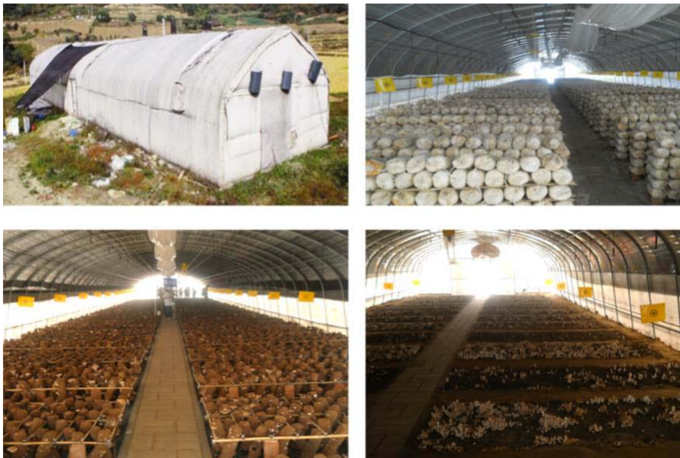
Fig. 5. Mushroom polyhouse structures in China
