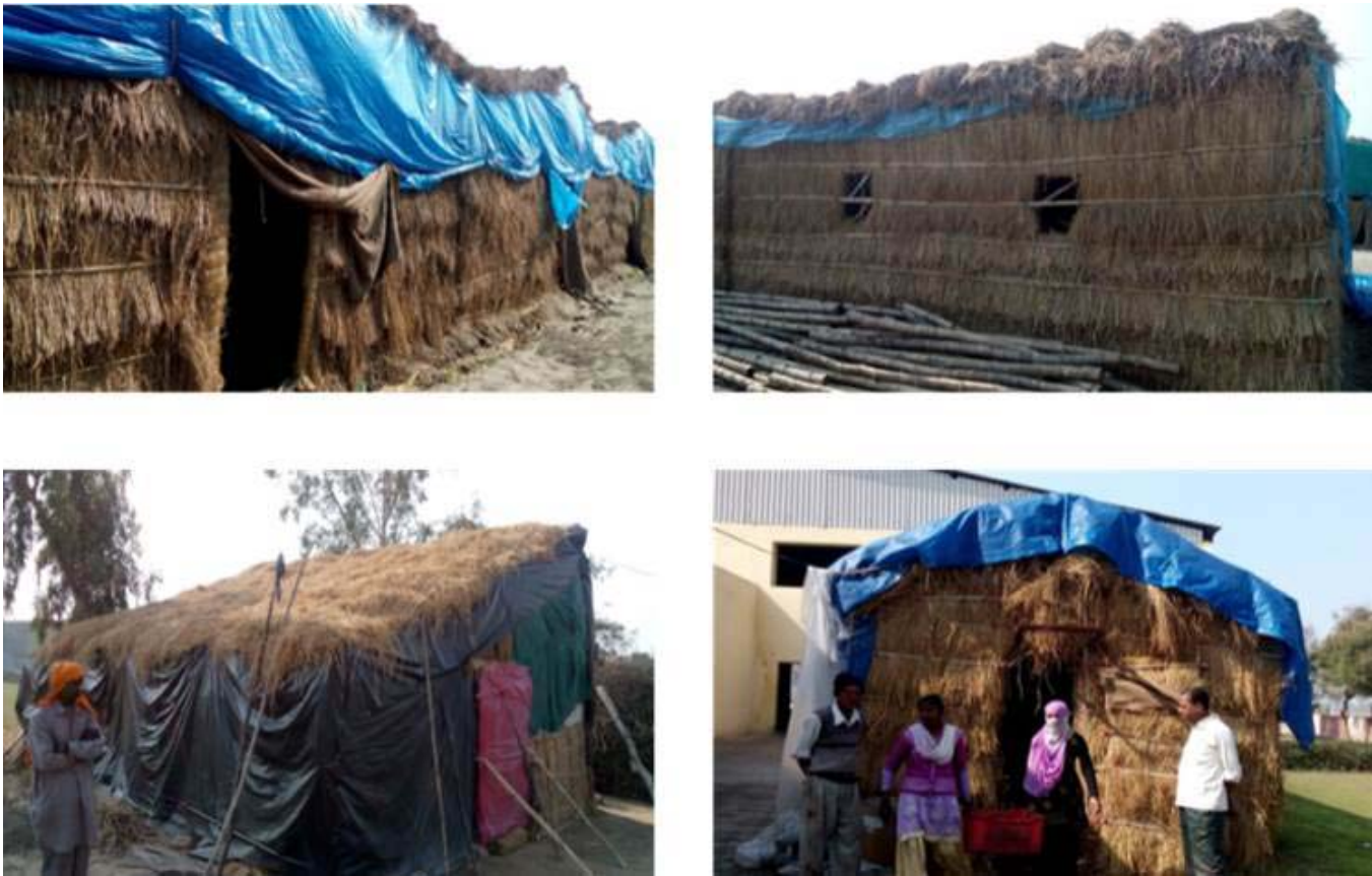
Fig. 2. Structures from locally available agricultural materials in Haryana and Punjab (Photo courtesy: S. J. Kale)
