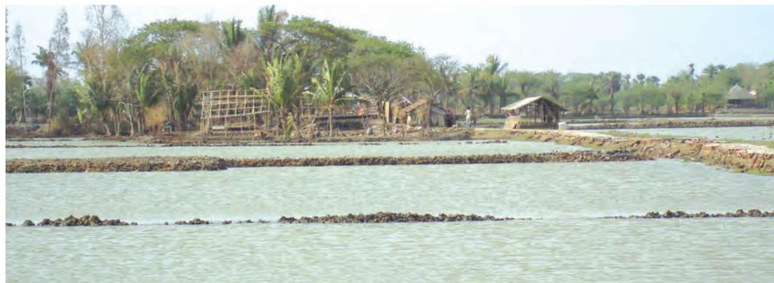
Inundation of ponds and infrastructure damage due to flood in Valsad dist., Gujarat
